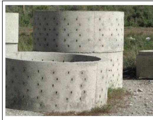
Figure E.4. Dry Well #1 – Structural Prefabricated Chamber.
